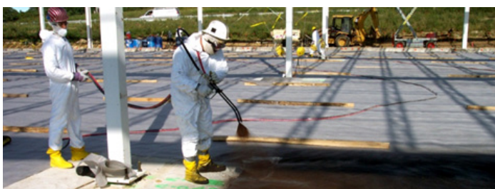
Figure 10. Geotextile fabric is placed over stone followed by spray application of the sealant.
