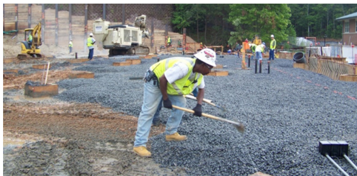
Figure 2. Proof-rolled ground covered with 8 inches AASHTO #57 stone.
