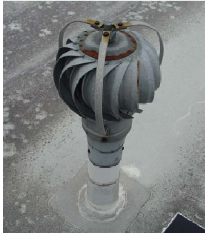
Figure 16. Roof vents fitted with wind turbines provide slight depressurization of the sub-slab area and prevent the buildup of contaminants beneath the building.
