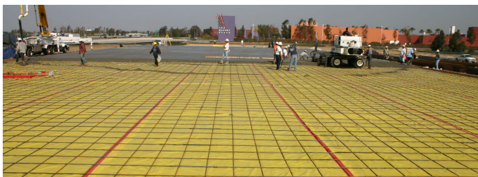
Figure 9. Polyolefin vapor barrier with sealed seams shown with rebar and concrete slab being installed over top.
