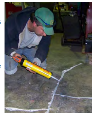
Figure 1. Sealing floor cracks.
