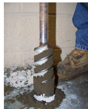
Figure 3. Suction point installation.
