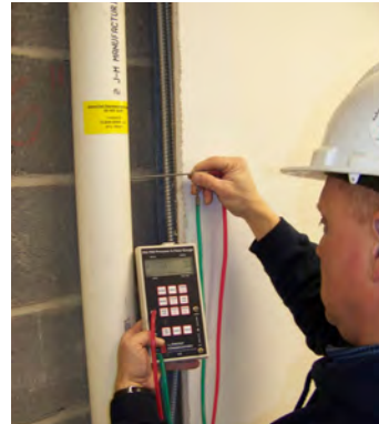
Figure 8. Riser pipe airflow test.
