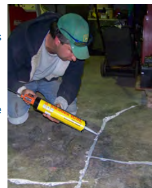
Figure 1. Sealing floor cracks.
