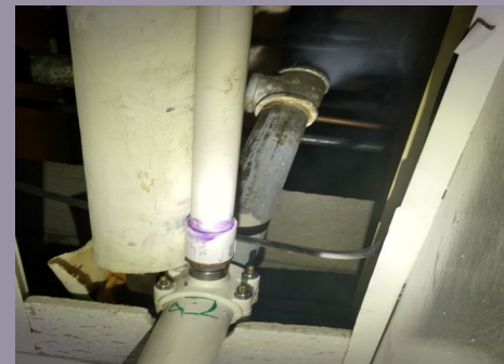
Sanitary Sewer Line Above Suspended Ceiling
