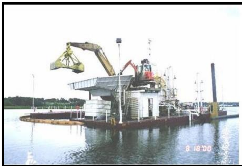
Figure 4-10. Hybrid Dredging System Used in New Bedford Harbor (Source: Battelle, 2010)
