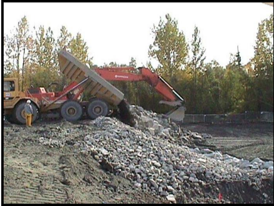
Figure 5-6. Armoring the Side of a CDF (Source: Battelle, 2010)
