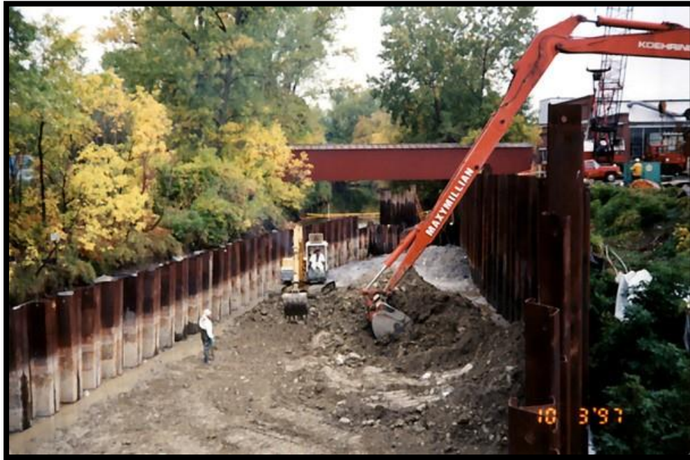
Figure 4-14. Excavation inside Cofferdams (Source: Battelle, 2010)
