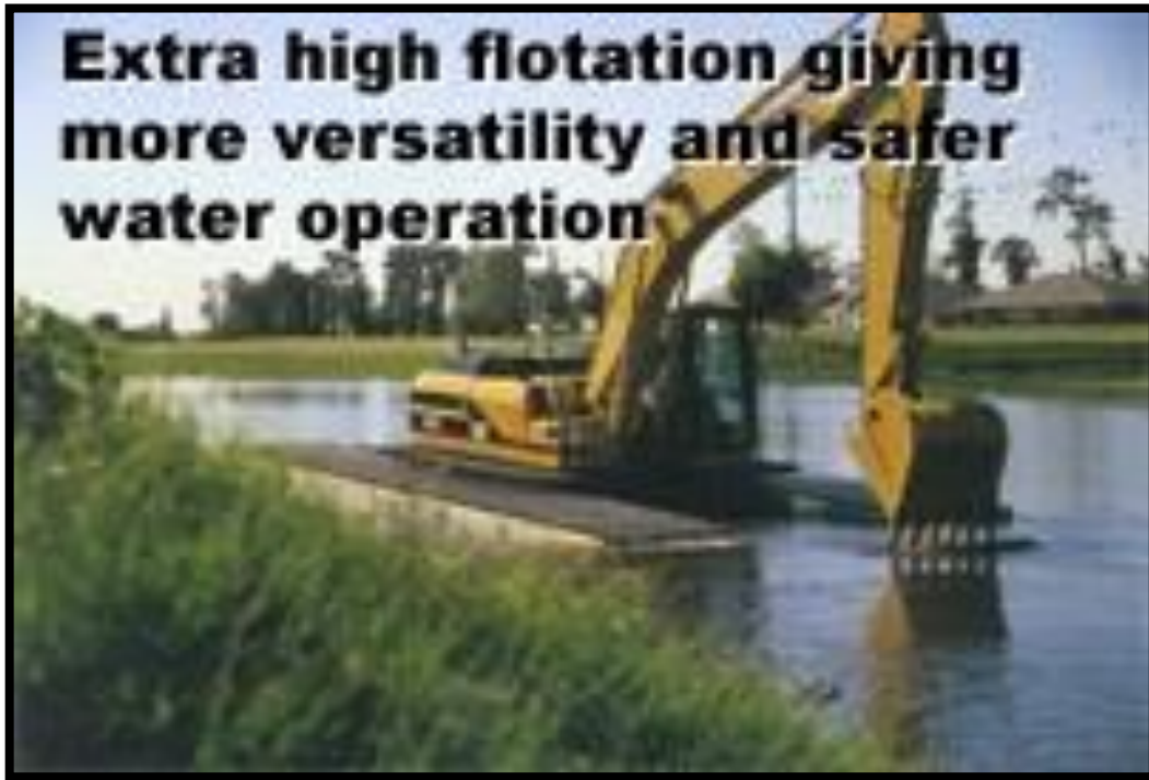
Figure 4-11. Floating Amphibious Dredge (Source: Battelle, 2010)
