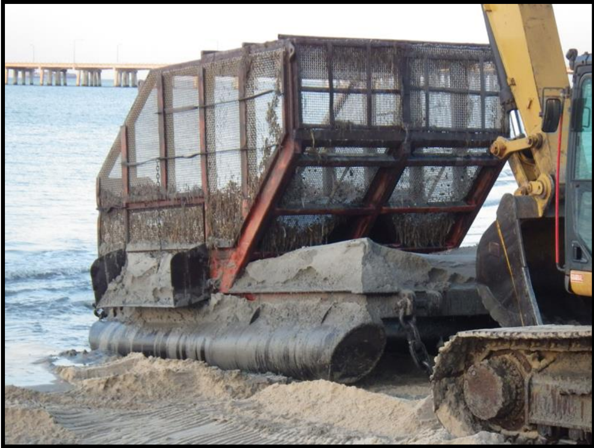
Figure 6-4. MEC/MPPEH Screening Basket, Chesapeake Beach, Virginia (Source: OHI)
