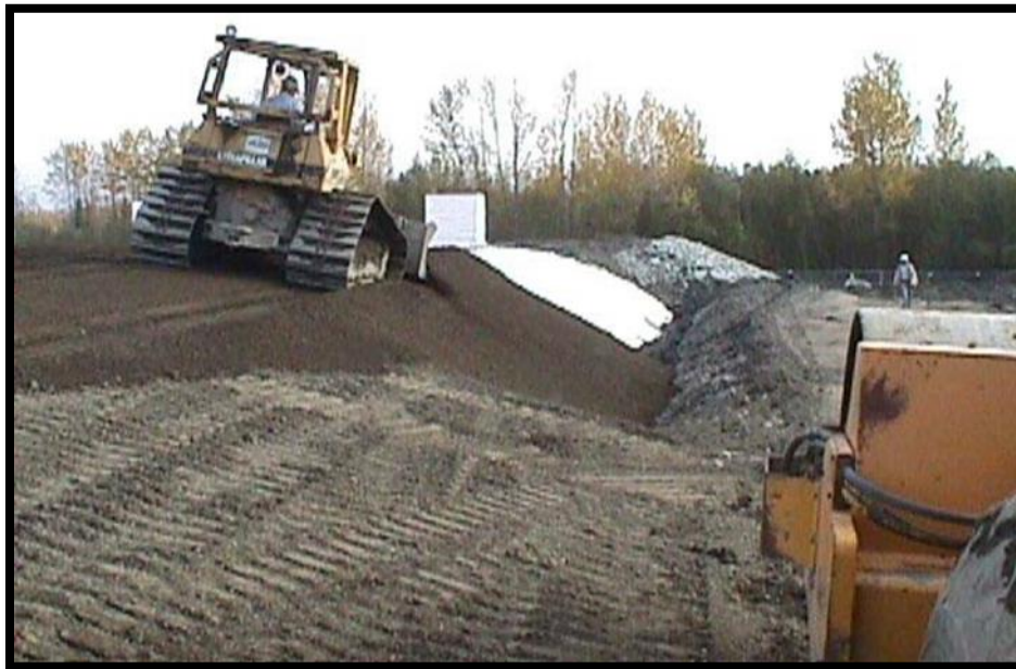
Figure 5-5. Grading the Side of a CDF (Source: Battelle, 2010)
