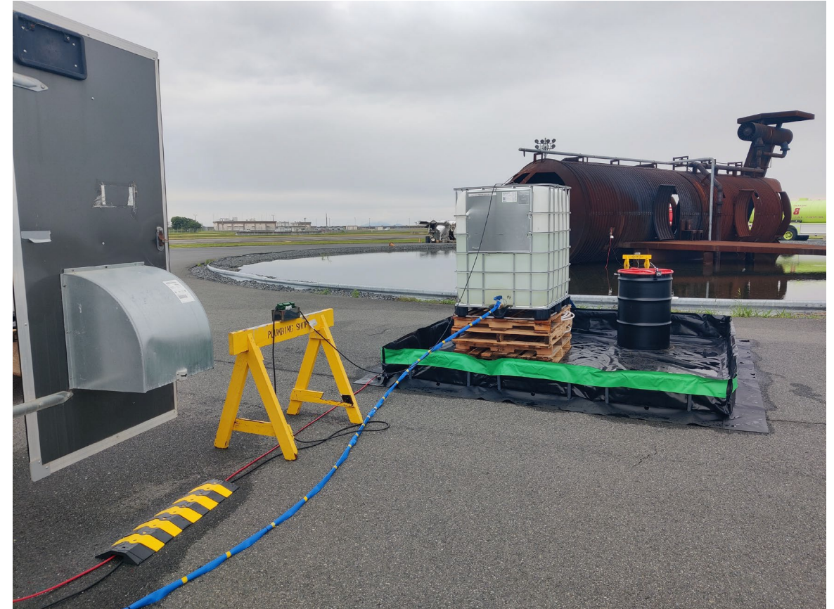
Influent ballast tank at Site 1 (Kornuc 2024)
