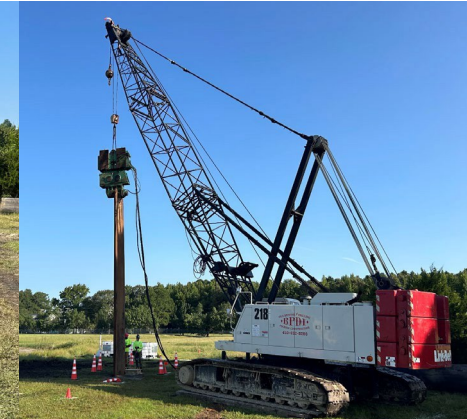
Sheet Pile Installation
