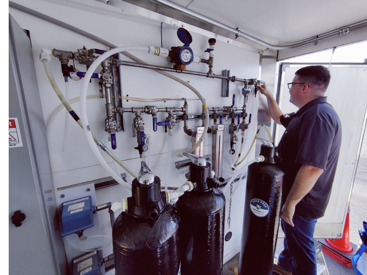
Change-out of GAC to cyclodextrin sorbent (Dexsorb canisters)
