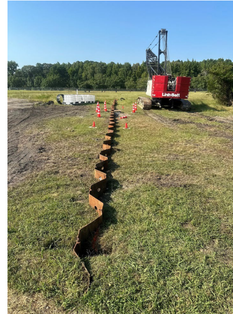
Sheet Pile Installation
