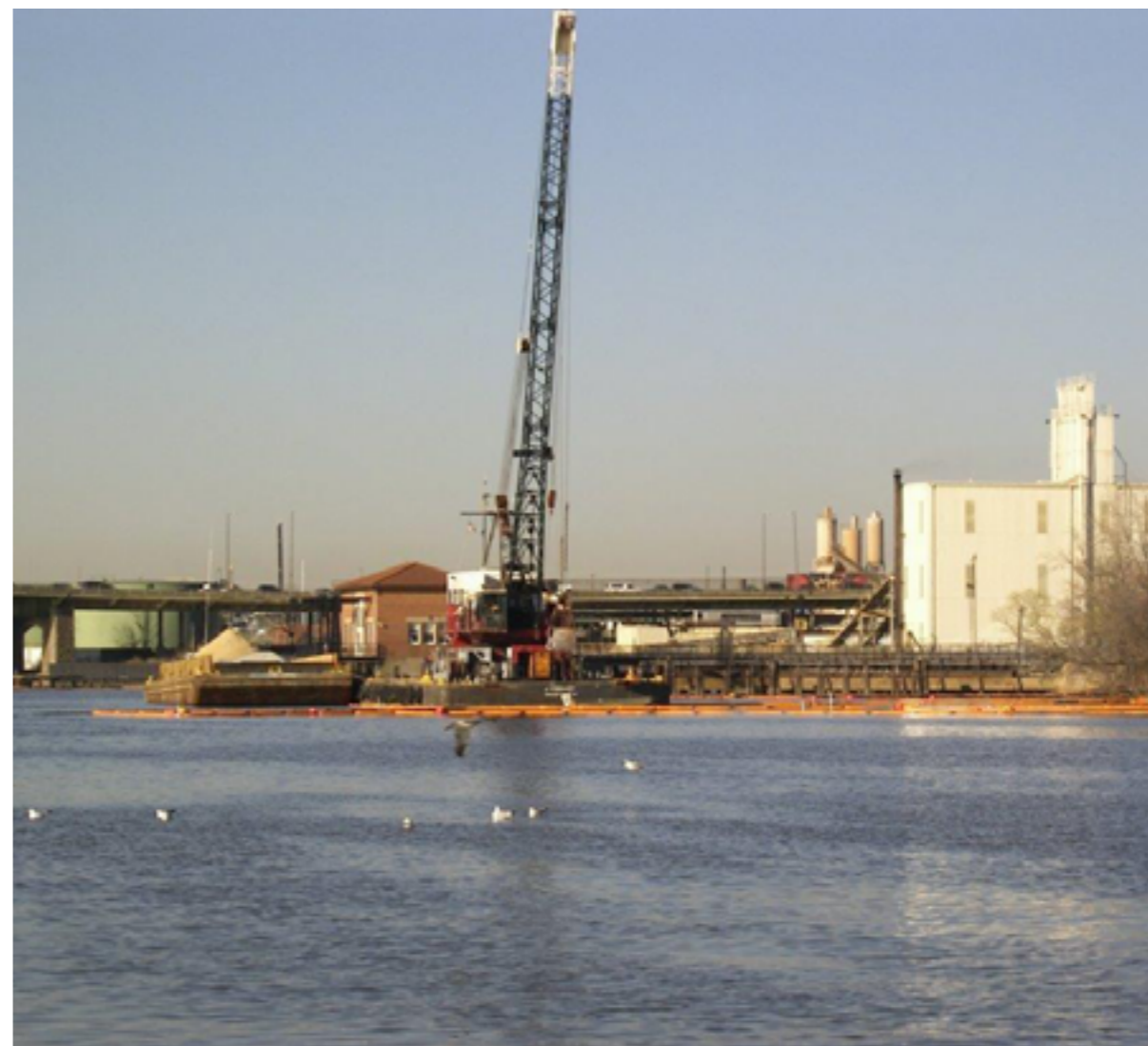
Figure 1. Reactive Capping for Contaminated Sediments
