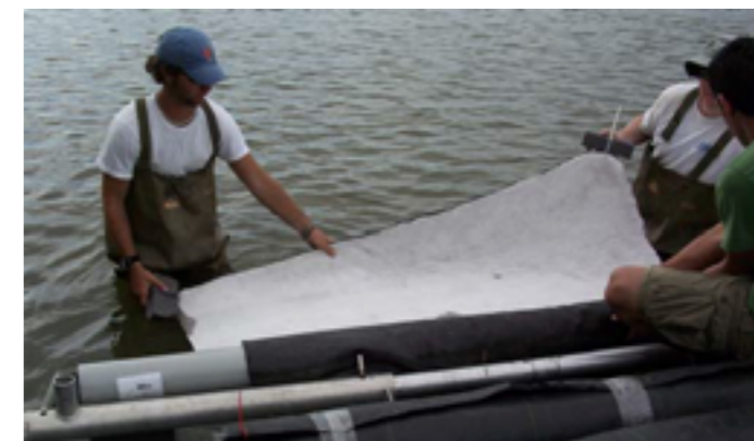
Figure 11. Small-scale geotextile test mat deployment.
