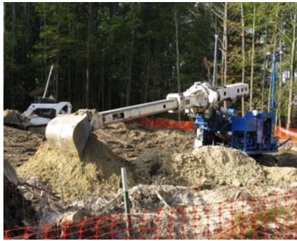
Remotely-operated subsurface MEC removal. Photo courtesy of US Navy.
