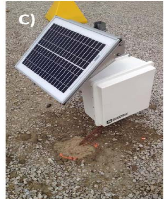
Solar power supply and weatherproof box with data logger and wireless communications system.
