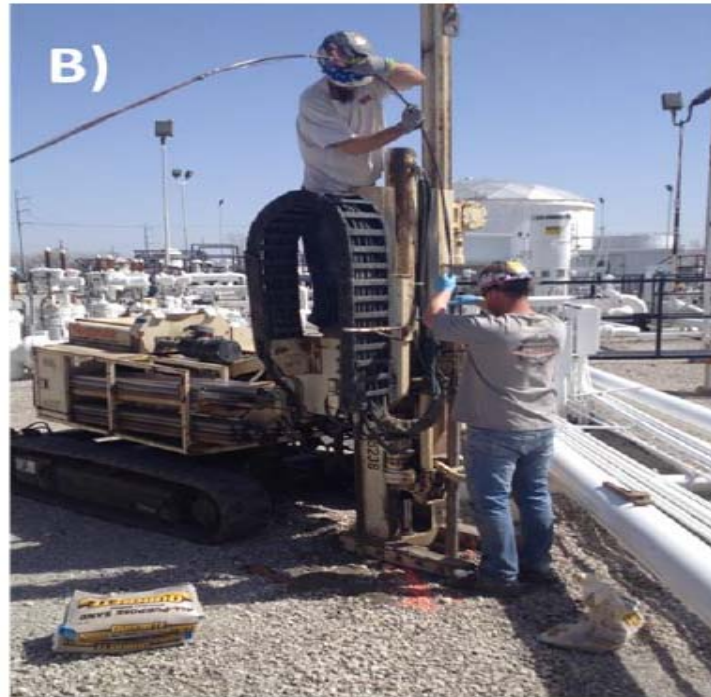
Installation of stick using direct push rig.
