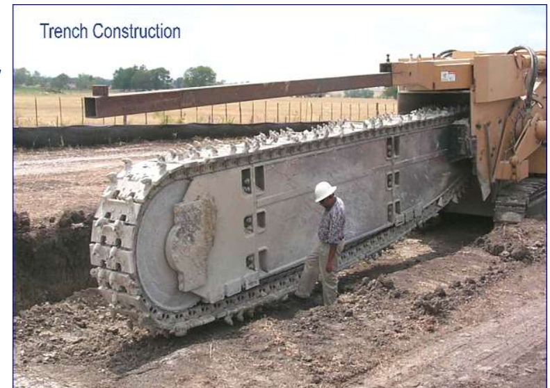
Trench excavator used to construct groundwater collection trenches
