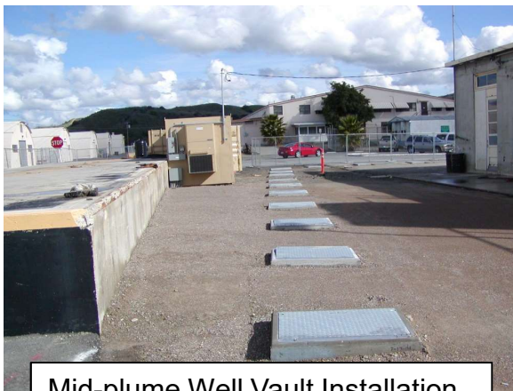
Mid-plume Well Vault Installation
