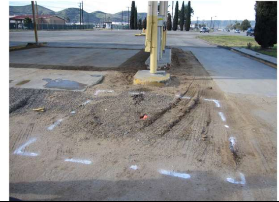
MGS source area prior to excavation
