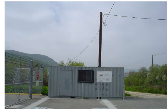
Leading-edge Oxygen Injection Biobarrier System
