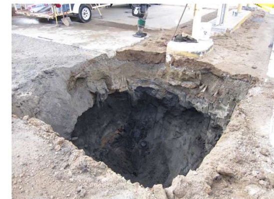
MGS source area excavation
