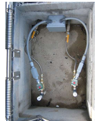
Oxygen Injection Wells in Vault
