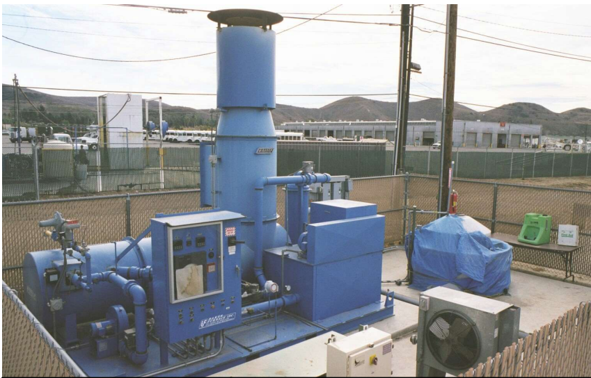
Primary MGS SVE/AS System with Thermal Oxidation
