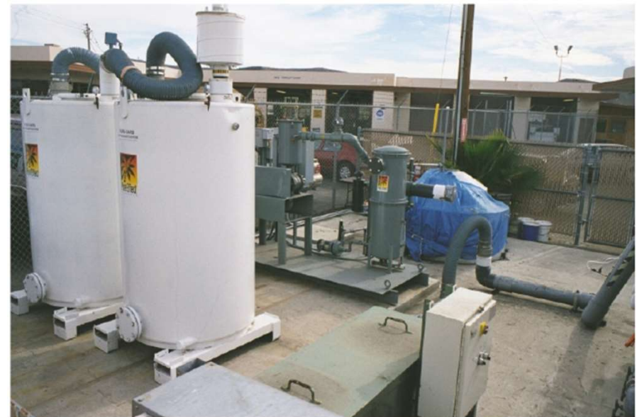
Primary MCX SVE/AS System with Carbon Filters
