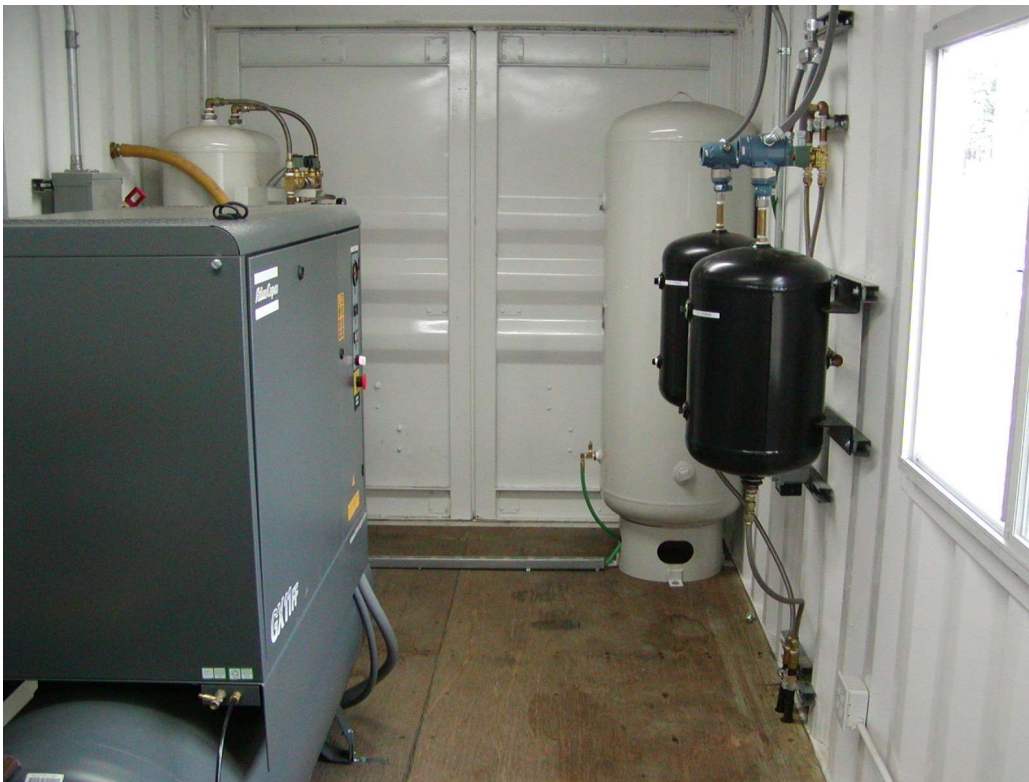
Compressor and oxygen holding tanks
