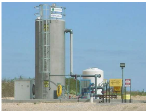
Fluidized bed reactor used for biological treatment of perchlorate (NAVFAC 2017)
