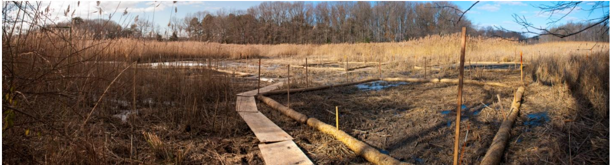
Figure 5-2 Cleared Test Plots, Staked Sediment Control Products, and Temporary Walkways
