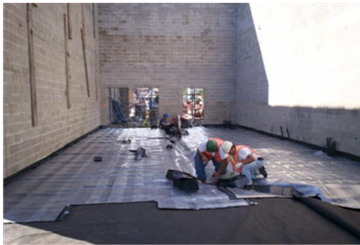
Figure 14-4. Passive Vapor Barrier Installation (Source: DON, 2010)
