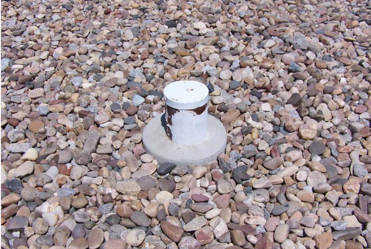
Figure 12-2. Settlement Monument (Source: UMTRC Annual Report, Maybell, Colorado, U.S. DOE, 2006 )
