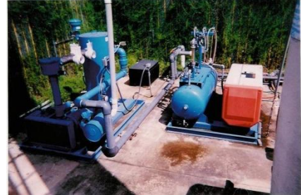
Air sparging uses air to help remove chemical vapors from both soil and groundwater. The soil vapor extraction system then works like a vacuum to extract and collect the volatile chemicals for proper disposal. AS/SVE systems work best on volatile chemicals, like those found at NWIRP, Site 1 - Former Drum Marshalling Area.
