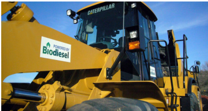
Soil Excavation using Biodiesel-Powered Equipment (EPA, 2008)
