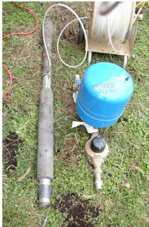
Figure 5.32. Packer, Pressure Tank and Water Meter Used During the Borehole Pressure Test
