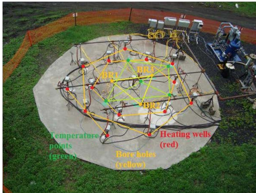
Figure 1 – Photograph of the TCH pilot-system installed for the source zone remediation of TCE at the NAWC site, including a diagram indicating the location of the heating wells, temperature measurement points and bore holes for core sample collection.
