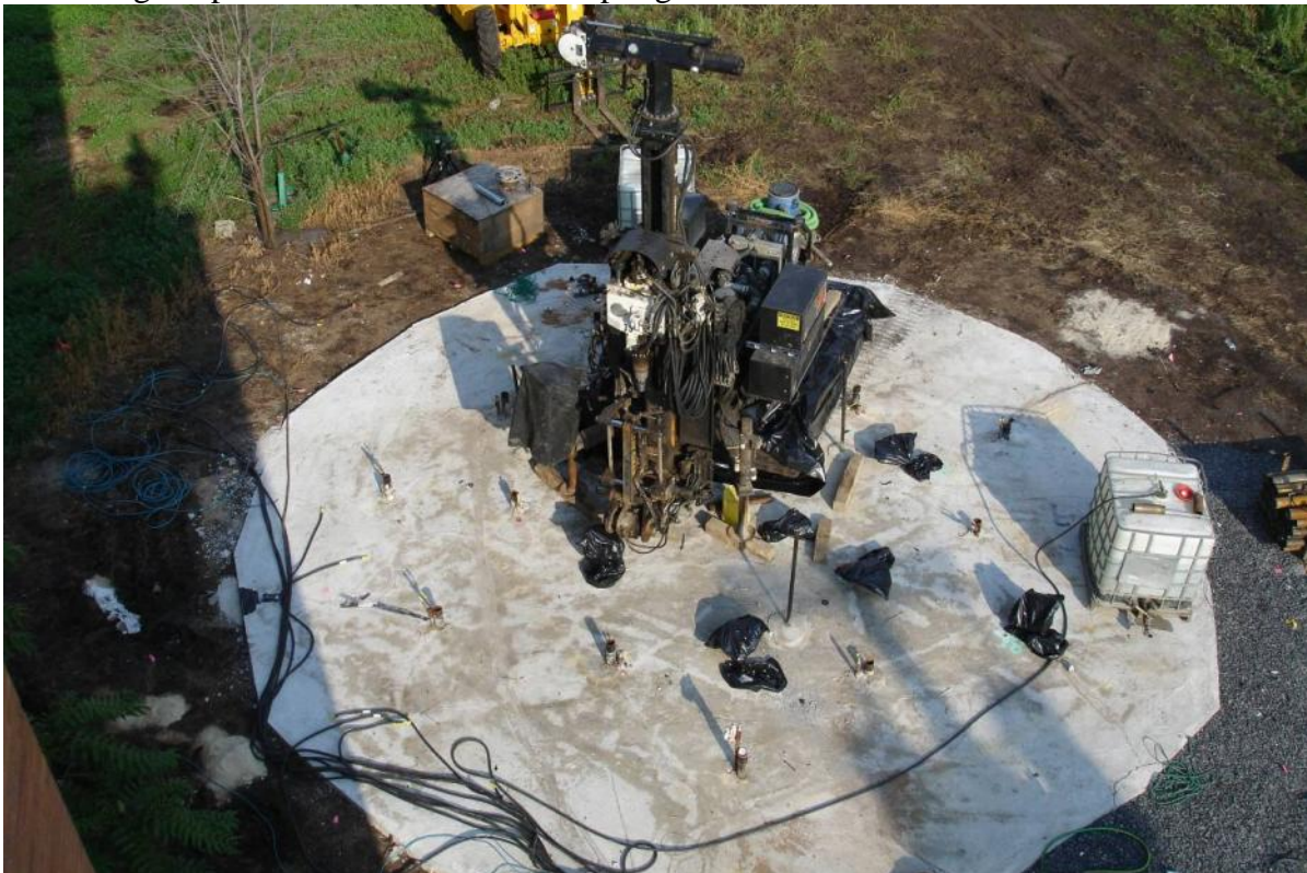
Figure 5.26. Drill Rig on Vapor Cap during Post-Treatment Bedrock Sampling
