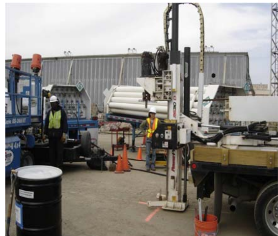
Figure 3-3. PFI Pneumatic Injection Equipment Layout
