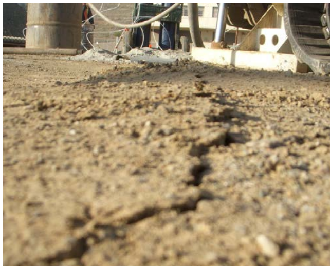
Figure 4-7. Surface Fracture and Uplift Formed during Pneumatic Injection of ZVI
