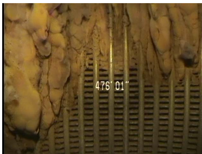
Figure 4-9. Fouling in a Deep Recovery Well
