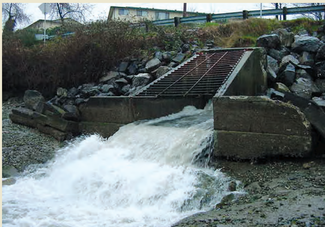
Stormwater outfall.
