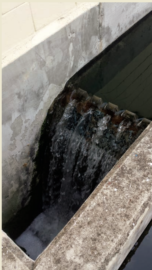
Outfall for the same wastewater treatment plant. The treated wastewater effluent discharges into a combined sewer line after chlorination.
