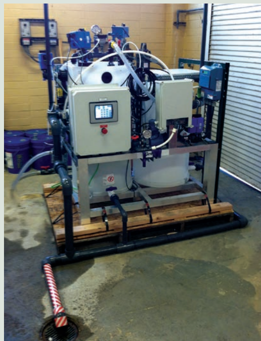
Skid-mounted mixed-metal treatment field unit at NAS Lemoore. Photo courtesy of CB&I Federal Services
