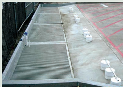
The dual media filtration system. Dual media chambers are shown on the left and float valves are shown on the right. Photo by Gary Anguiano
