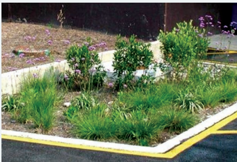
This bioretention planter helps minimize stormwater runoff.
