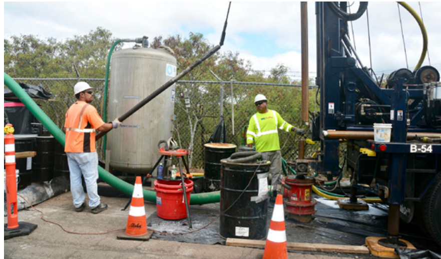
Soil and/or wastewater from well installations can be a source of per and polyfluoroalkyl substances. (Photo Credit: Theanne Tangen)
