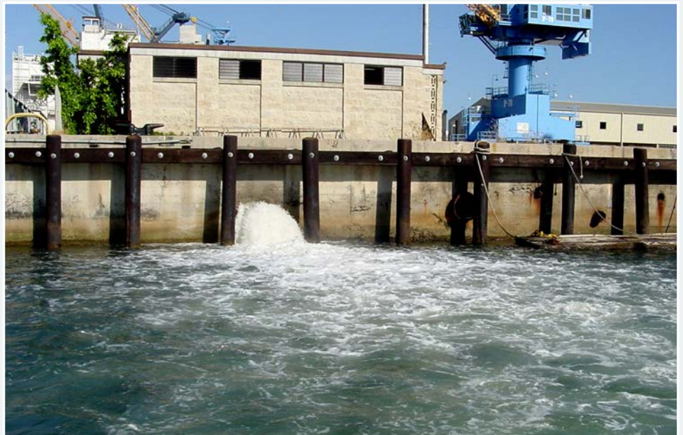
Stormwater outfall.
