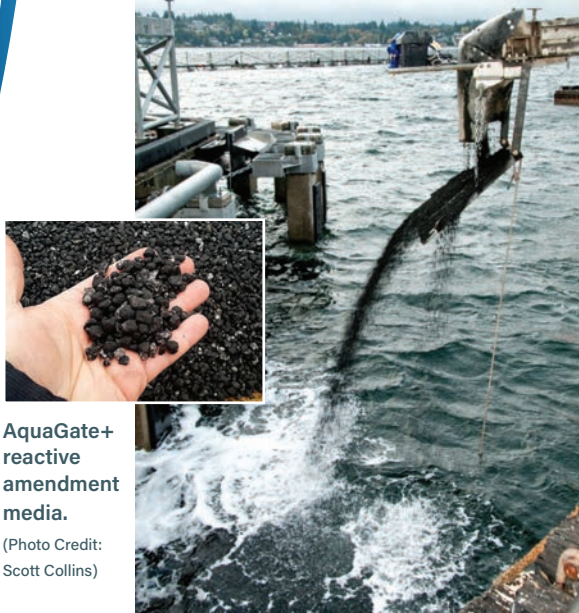
AquaGate+ amendments being deployed at a Navy site. (Photo Credit: Courtesy of ESTCP project no. ER-201131)
