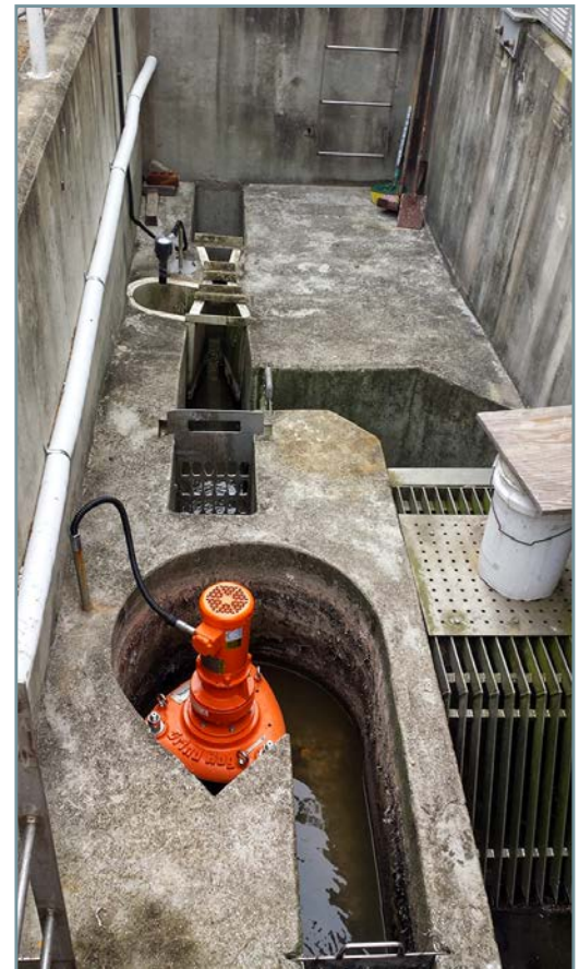
This wastewater treatment plant is designed for an average daily flow of 107,000 gallons per day. This image was taken during a time of low flow into the plant and shows the incoming sewage flowing through two bar screens, and finally into a Parshall flume where the flowmeter records the flowrate of the influent wastewater. (Photo Credit: Tami Relph)
