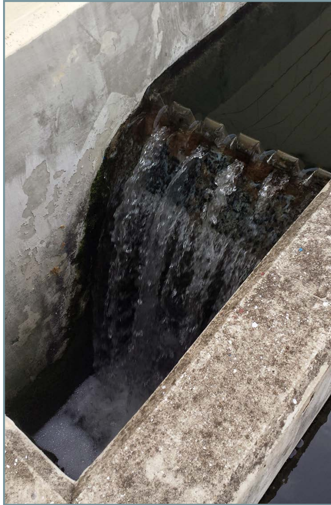
Outfall for the same wastewater treatment plant. The treated wastewater effluent discharges into a combined sewer line after chlorination.
