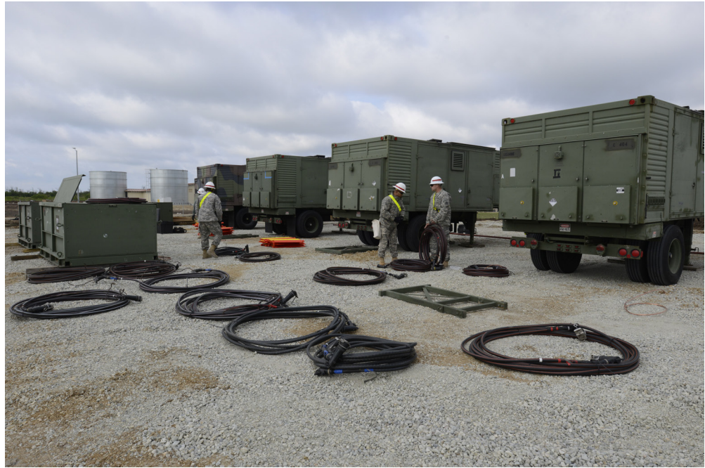
Forward deployed portable generators require tracking and monitoring of routine maintenance, operating time and time-in-location. (U.S. Navy photo by Lt. Cmdr. Mike Billips)
