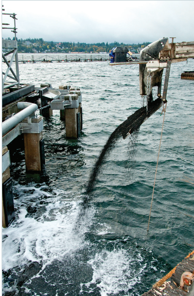
AquaGate+ amendments being deployed at a Navy site.
