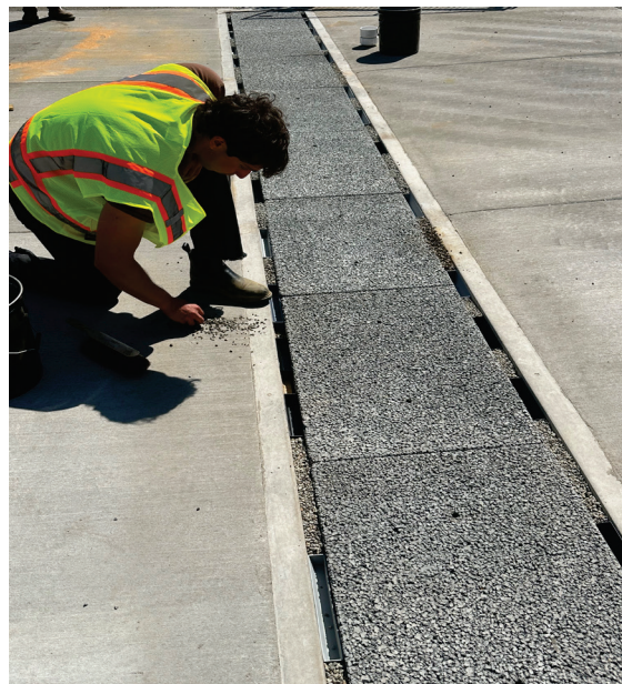
Installation of LIPPS at PSNS for the capture and treatment of stormwater runoff. (Photo credit: Denis Acosta)
