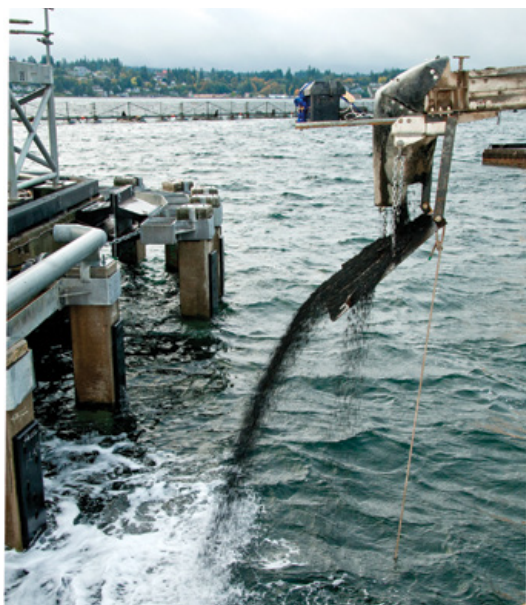
AquaGate+ amendments being deployed at a Navy site. (Photo Credit: Courtesy of ESTCP project no. ER-201131)
