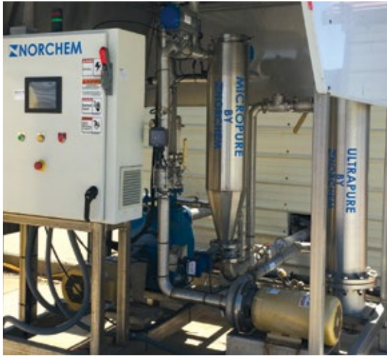
This dissolved air technology is being demonstrated to mitigate toxic gases from sanitary sewers onboard NAB Coronado. (Photo Credit: Steve Fann)
