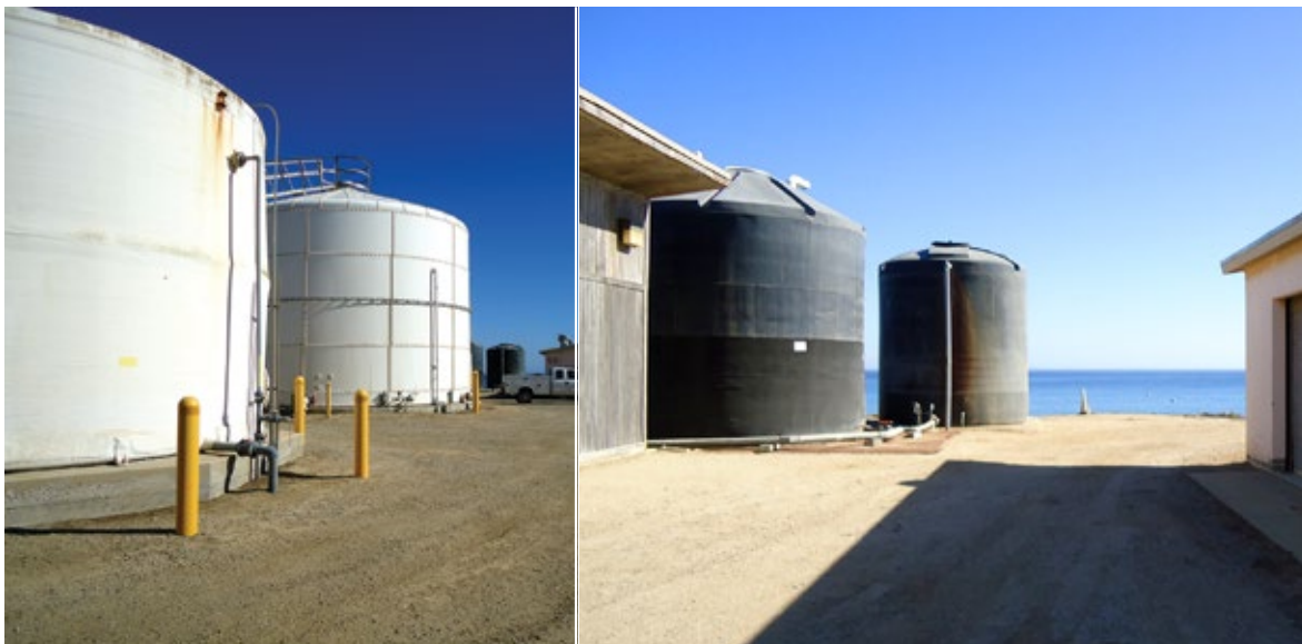
Navy drinking water treatment facility with potable treated water storage tanks and reverse osmosis tanks. (Photo Credit: Autumn Resto)
