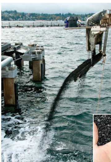
AquaGate+ amendments being deployed at a Navy site. (Photo Credit: Courtesy of ESTCP project no. ER-201131)
