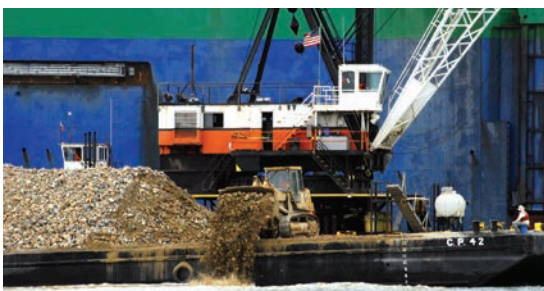
A barge distributes tons of armored rock on top of a confined aquatic disposal cell. This IDR will provide a comprehensive strategy to guide the NESDI program's investments in the Navy's contaminated sediment management area. Photo Credit: Vance Vasquez
