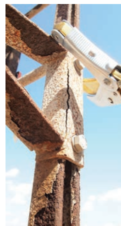
Heavy corrosion and coatings failure on galvanized tower.
