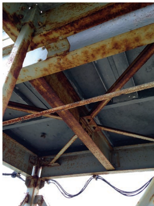
Corrosion on underside of galvanized tower related to exposure to salt spray.
