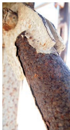
Close-up of corrosion on coated, galvanized structure.
