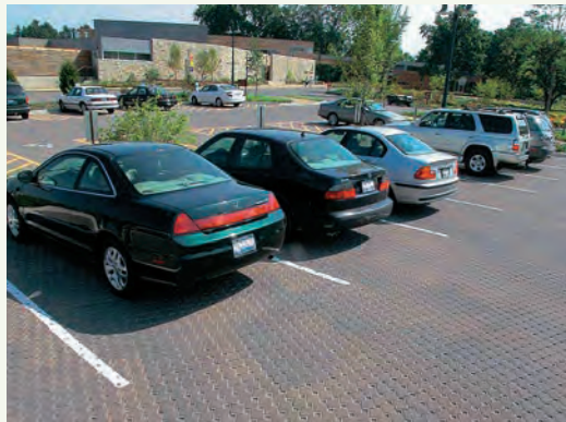
The use of porous pavers is one example of low impact development. (Photo Credit: Chuck Katz)
