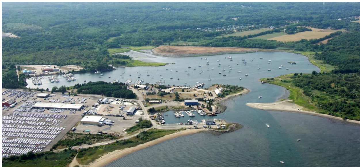
Figure 2. Aerial view looking west into Allen Harbor and the entrance channel. The former Naval Construction Battalion Center (NCBC) Davisville Site 7, in North Kingstown, Rhode Island, was on Calf Pasture Point (on right). (Source: https://marinas.com/view/harbor/75t61_Allen_Harbor_Allen_Harbor_RI_United_States )
