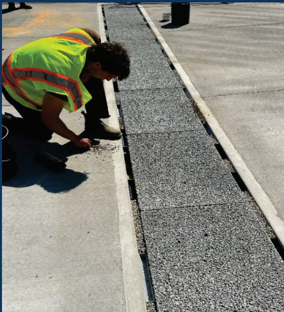
Installation of LIPPS at PSNS for the capture and treatment of stormwater runoff – NESDI Project 583. (Photo credit: Denis Acosta)
