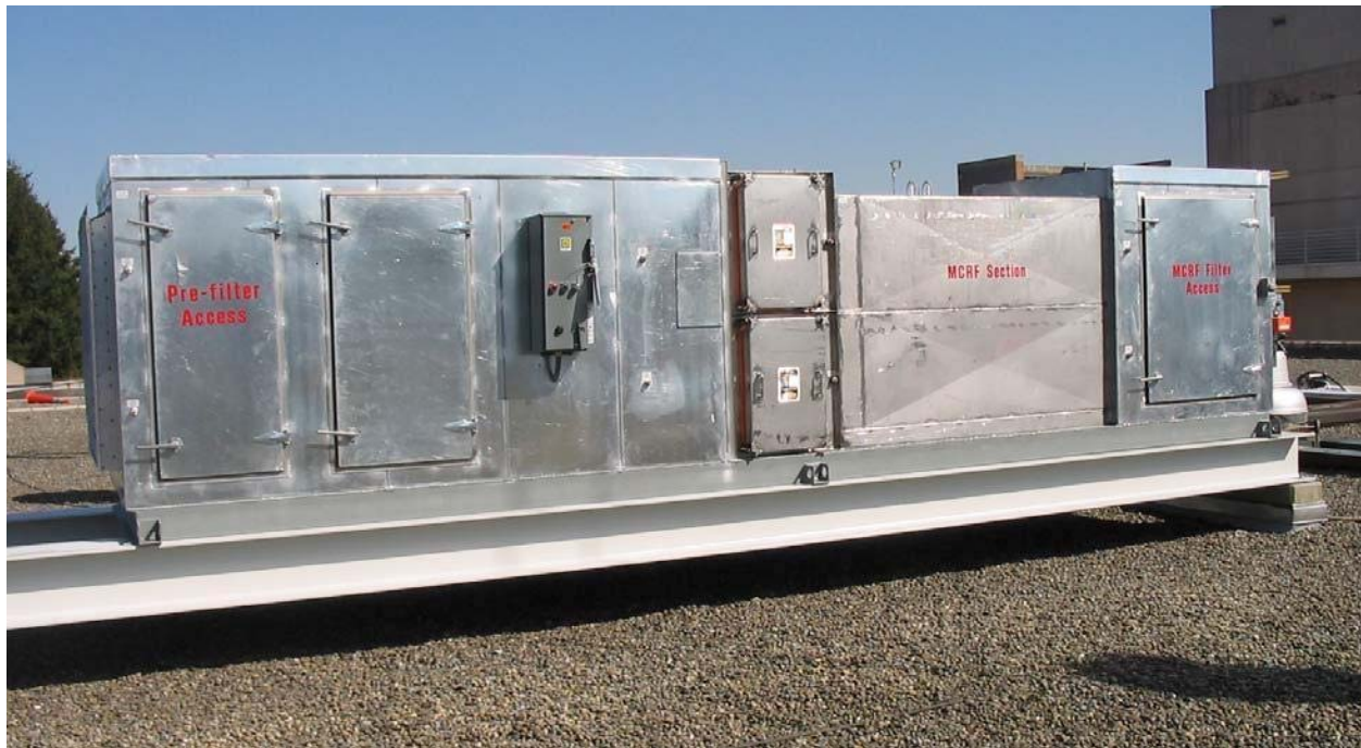
Figure G-12. Multi-Cell Radial-Flow (MCRF) Filtration Unit
