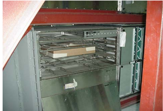
Figure G-6. Two 1,200-cfm M49 Assemblies Installed with HEPA Filters and Prefilters
