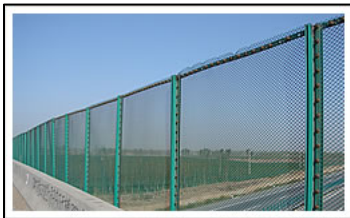
Figure 2-4: Expanded Metal Fence
