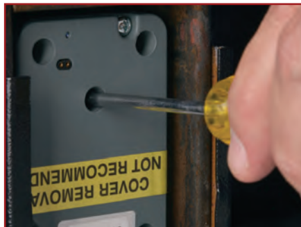
Figure 9. Tightening Spindle Screw
