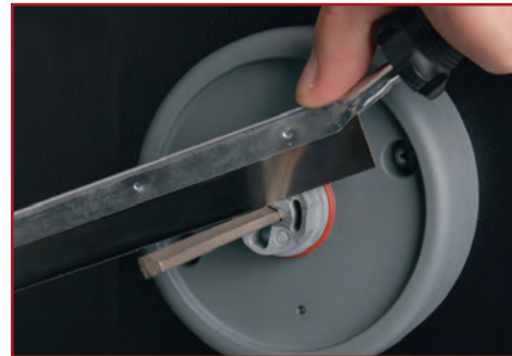
Figure 8. Cutting off Excess Spindle Using Hacksaw
