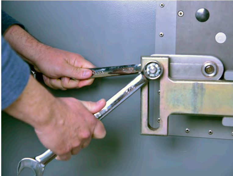
Figure 5-2. Removal of Castle Nut
