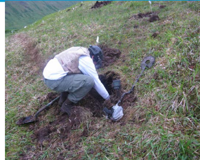
UXO Technician detecting and removing subsurface anomalies.
